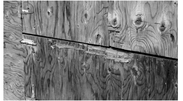
Shown above are the damages made by the bears on the old wooden garbage bin.
