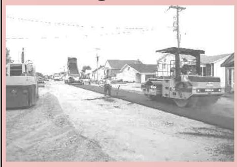
Work crews install new asphalt on a stretch of Lansdown in a realignment measure. The fix was ordered by the Township of Chapleau and the cost was assumed by the engineering firm, Kresin Engineering of Sault St. Marie. The original work was a part of the Lansdown-Aberdeen project which brought updated municipal services to the residential neighbourhood. The new pavement was installed by Palmer Construction Group Inc., of Sault Ste. Marie.
