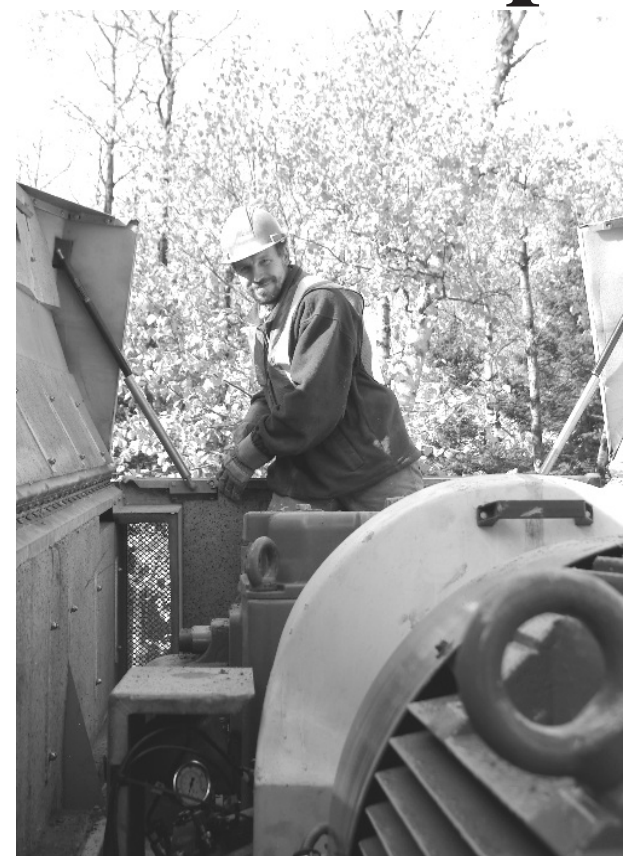
Yvon Martel making final adjustment to the access doors.
