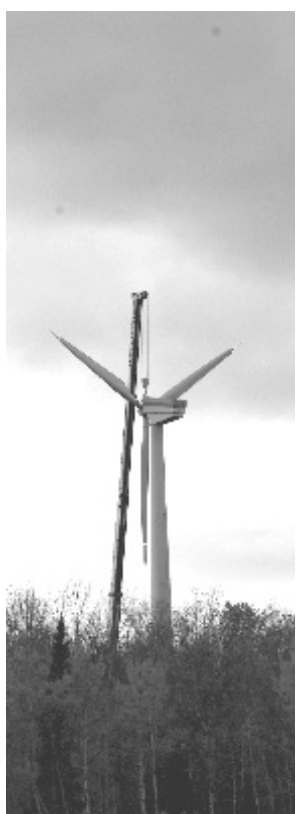
The crane puts final assembly up
