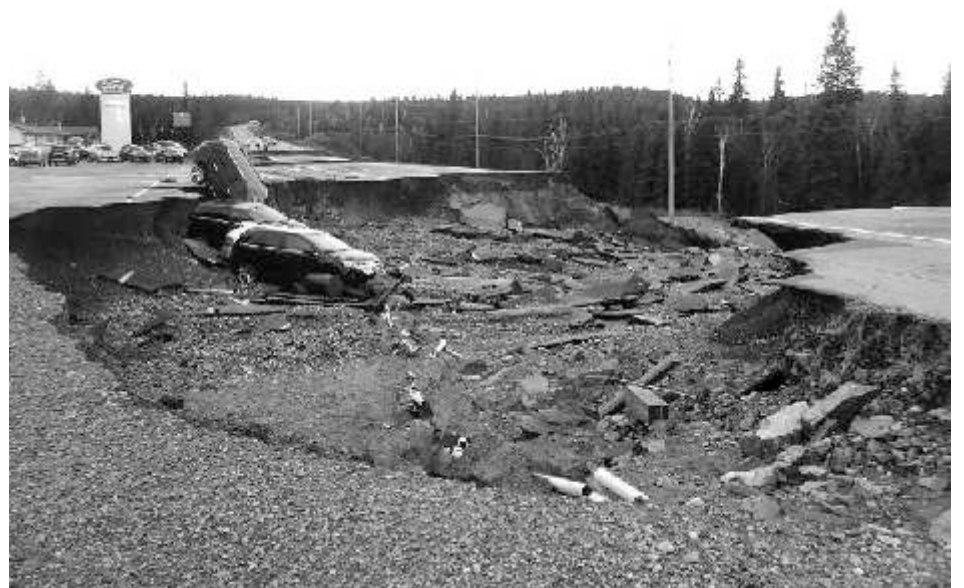
Shown above are vehicles belonging to Northern Lights Ford in the sink hole created by more than 130 mm of rain that fell in the area on Friday October 26th, 2012
