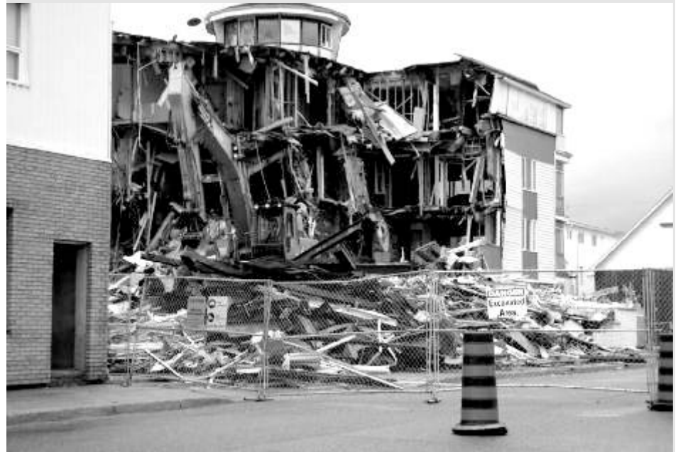
A few weeks ago the demolition of what was Dr. Young's apartments and offices was initiated. The building is now completely gone. Another landmark vanishing from the Chapleau landscape!
