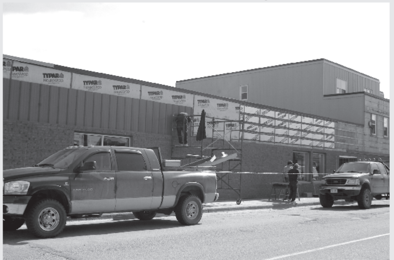
This week contractors were busy changing siding on our local hardware store, Collins Home Hardware. The bright red colors will certainly add to the already positive mood of the local townspeople.
