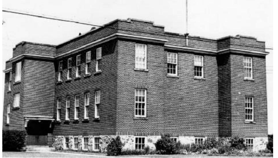
Chapleau High School on Pine Street
