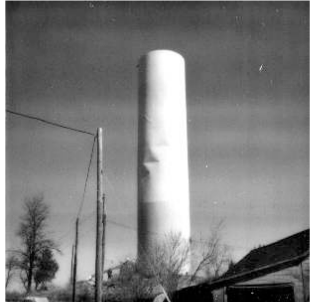
Dents in the water tank after it buckled inwards, April 1977
