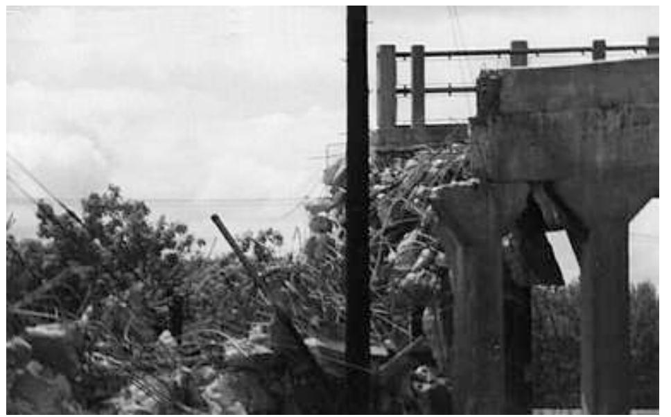
Demolition of old horseshoe bridge (from Dr. G.E. Young collection)
