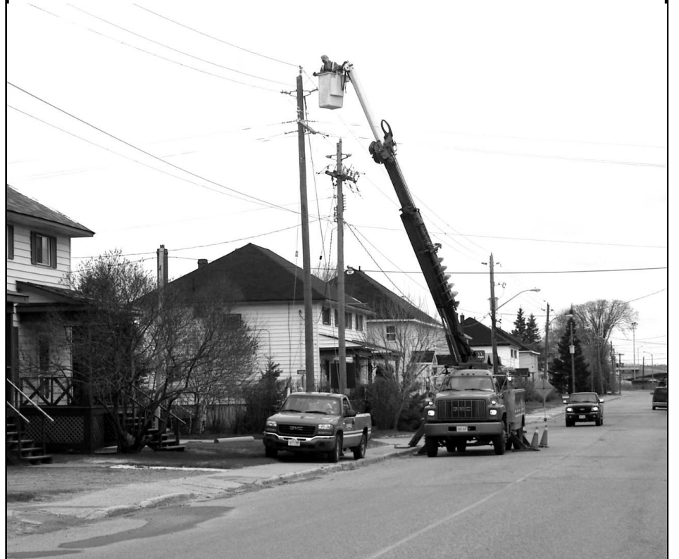
A power outage last Sunday was necessary for the Chapleau Public Utilities to move hydro poles to facilitate the re-routing of traffic for the upcoming Monk Street repair beginning later this month.
