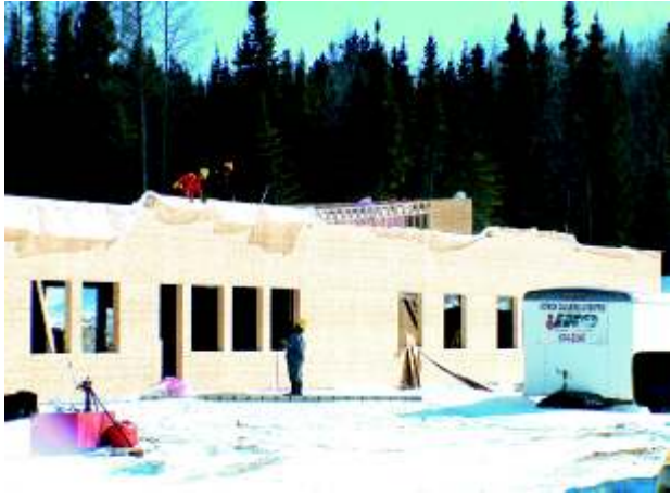
Construction crews finish the outside walls in preparation for the roofers.
