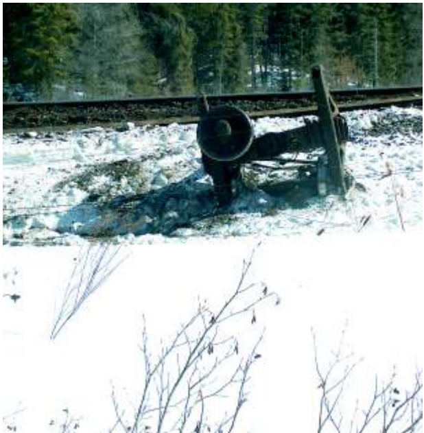
A set of wheels (trucks) from under a box car or tanker lay beside track which is twisted and mangled.
