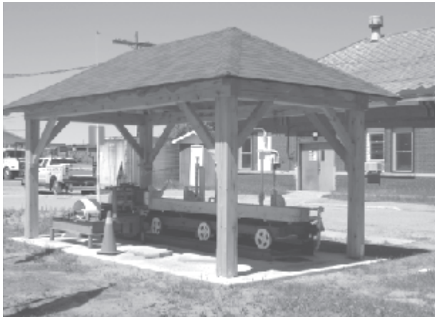
The newly completed structure covering the J.E. Martel replica sawmill.
