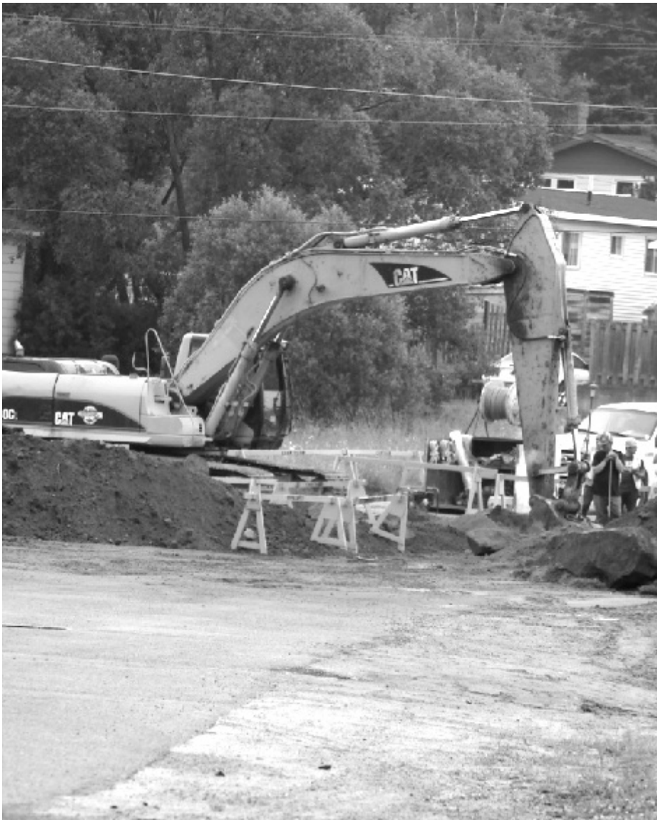
The ground was broken this week marking the beginning of water main and sewage line replacements on Devonshire and Cherry Street. Money was allotted earlier this year by the Ontario Government.
