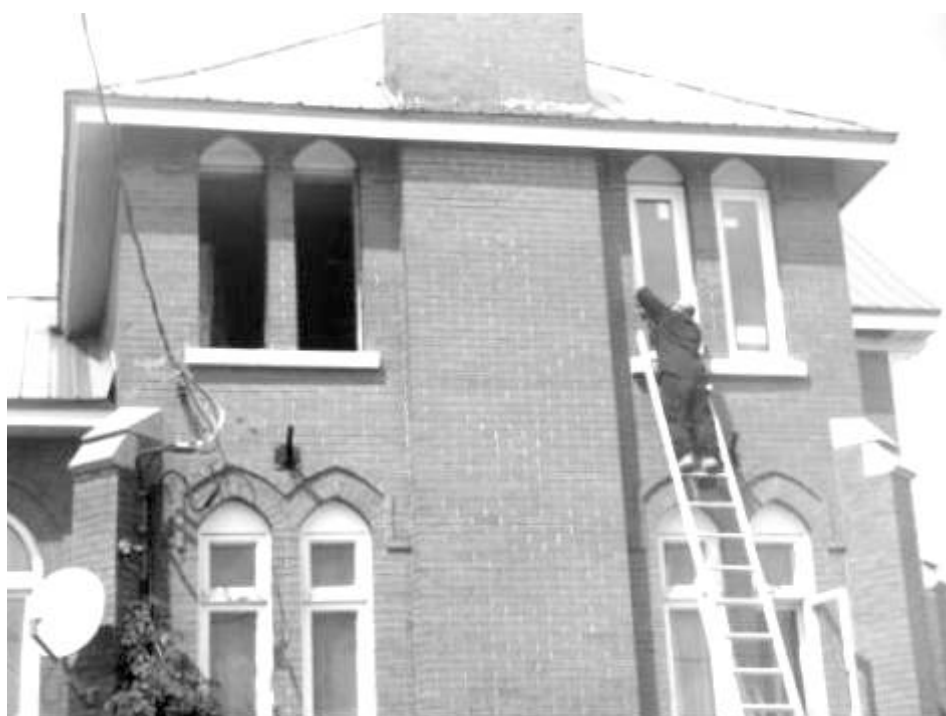
Bedard Contracting replacing windows at Legion
