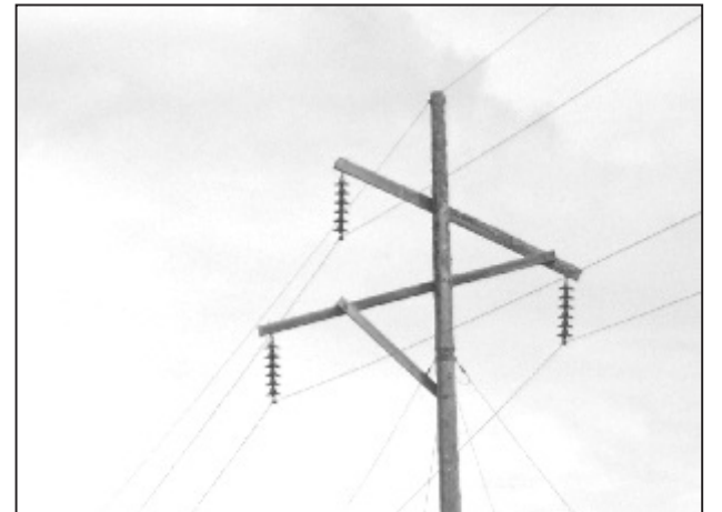
Traffic along highway 101 between Chapleau and Wawa is afforded a good view of the Hydro One line which brings electricity to Chapleau and Wawa. Aged wood cross arms are being replaced with metal fixtures to improve reliability of service to Chapleau customers.
