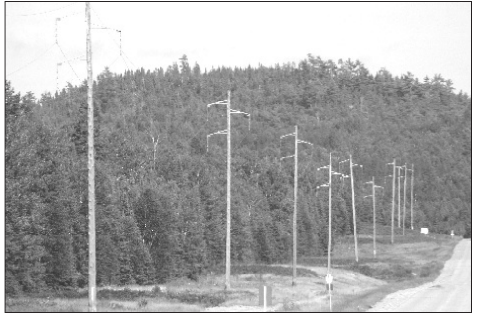
Traffic along highway 101 between Chapleau and Wawa is afforded a good view of the Hydro One line which brings electricity to Chapleau and Wawa. Aged wood cross arms are being replaced with metal fixtures to improve reliability of service to Chapleau customers.
