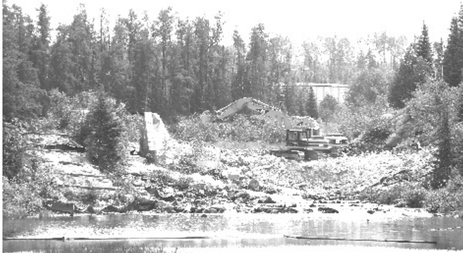
Nebskwashi River on highway 129 at entrance to Chapleau takes on a new look as historic dam has been removed.
